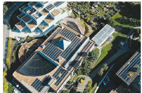
Photovoltaik-Anlage am Campus
