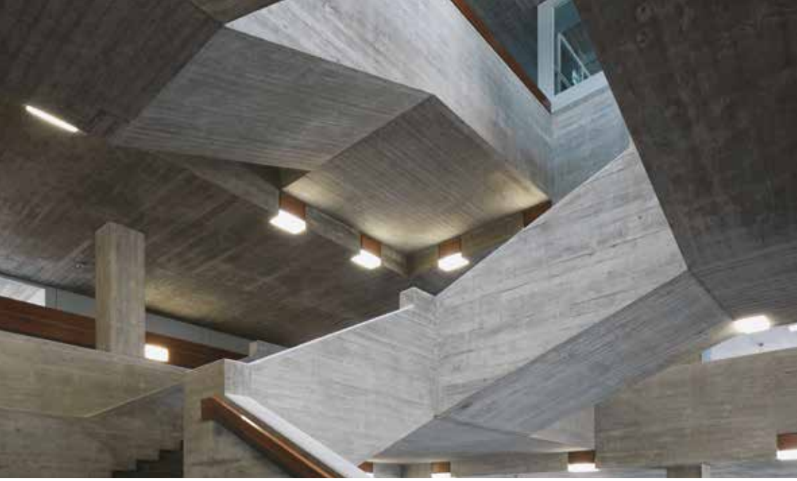
Imposing and sculptural. The self-supporting concrete staircase in the Main Building's great hall
